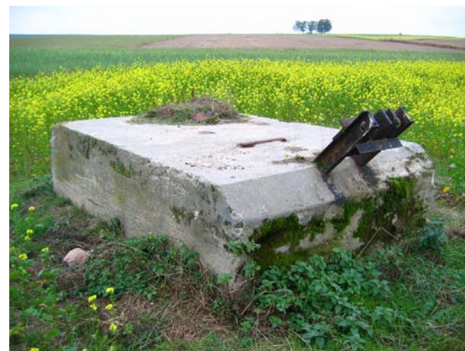
Anchor block, identical to that of M I/II.
